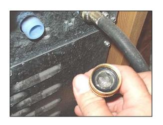
Remove water inlet hose filter screens to clean and replace if necessary.
