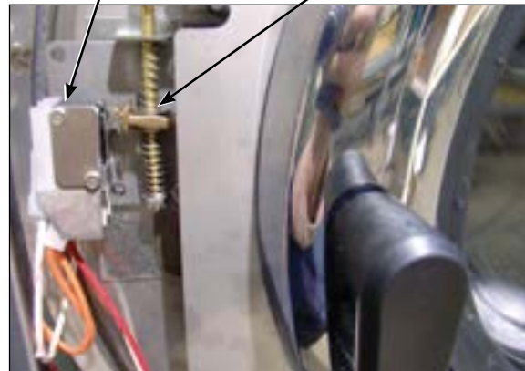
Adjustment screw for (piggyback switches) Top of flat end of locking pawl.
