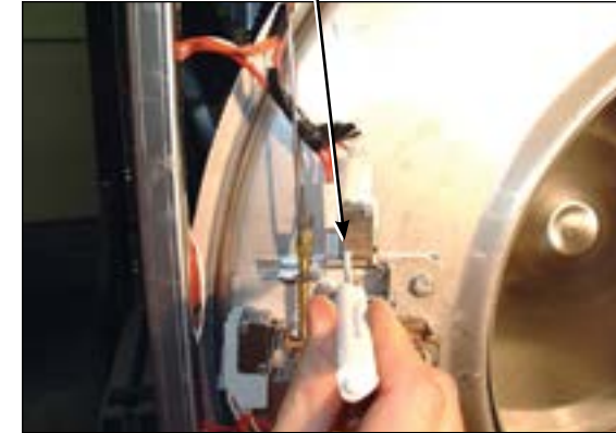
Flat blade screw on door switch latching
