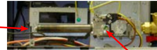
Adjustment Screw Under Plug
