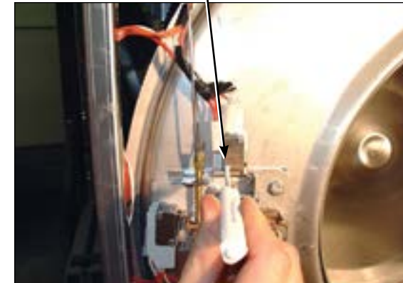
Flat blade screw on door switch latching
