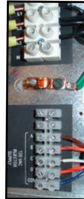
120VAC Injector Supply Connections Power Connections
