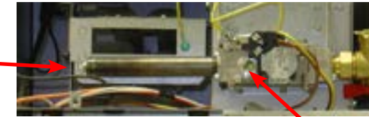
Adjustment Screw Under Plug
