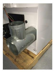
4) Install 9810-020-001 TEE ASSEMBLY – RECIRCULATION with (2) provided screw (if allowable by code) into the top.
