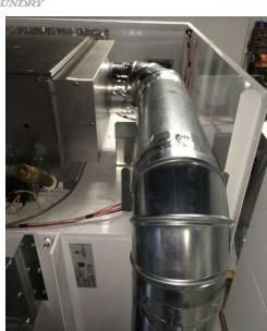
10) Finish upper joints with foil duct tape.
