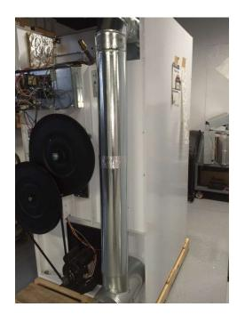
9) Install the duct from step 7 as shown and put (2) screws in the upper and lower joints.
