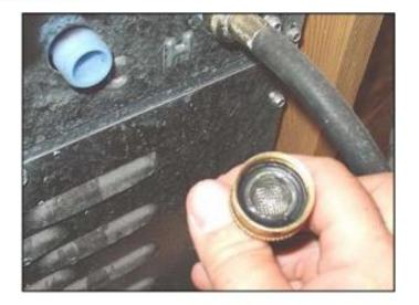
Remove water inlet hose filter screens to clean and replace if necessary.
